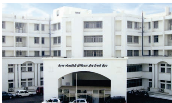
Terna Specialty Hospital & Research Centre
